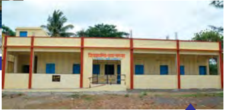
Salvad School : New Building
